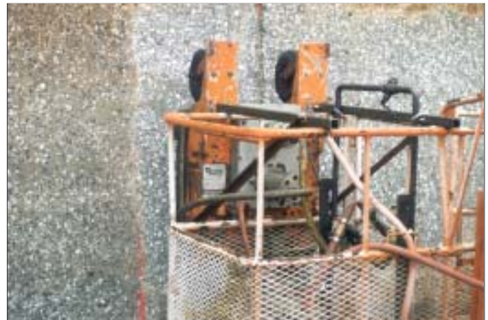
The NLB 20K Spin Jet is moved along the wall with a man lift, allowing for quick and efficient application of the high pressure water.
