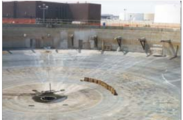
View of the concrete digester tank, midway through the cleaning process.
